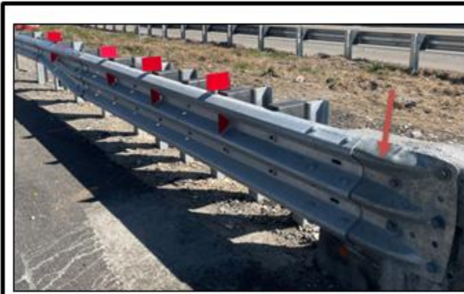
Example Photo of Bridge Connection - Long
