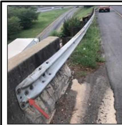
Example Photo of Bridge Connection – W Beam
