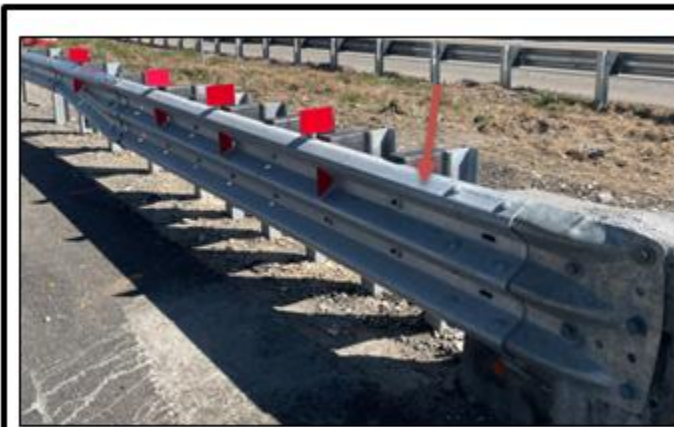
Example Photo of Bridge Connection - Long
