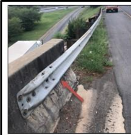
Example Photo of Bridge Connection – W Beam
