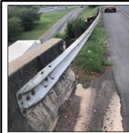
Example Photo of Bridge Connection – W Beam
