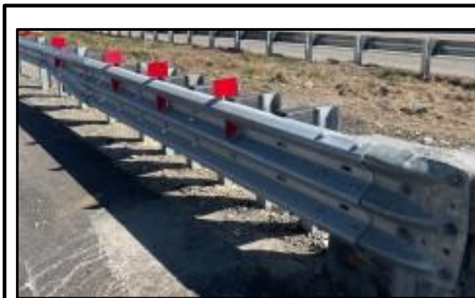
Bridge Connection - Long
