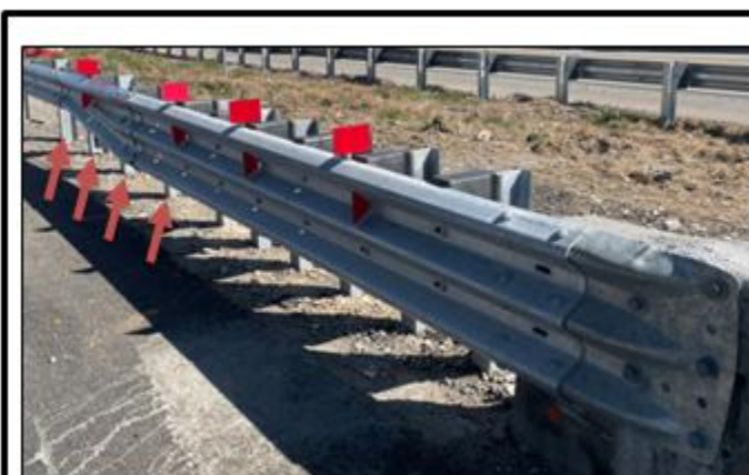
Example Photo of Bridge Connection - Long
